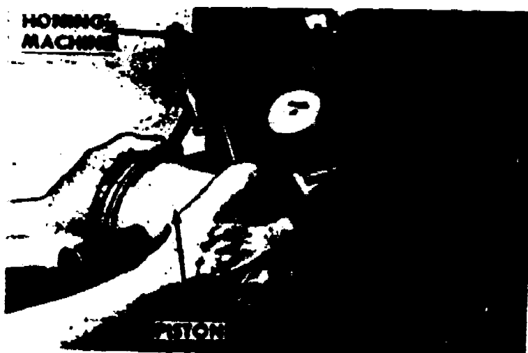
Figure 23. Honing Piston Pin Bosses.
