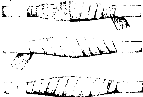
Figure 12-11.—Wrapping the splice.
