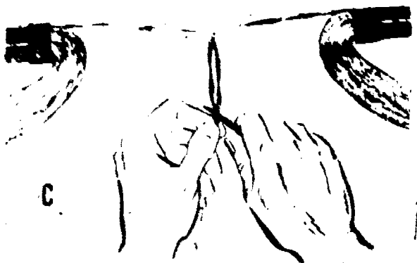
Figure 12-5.—Joining a pair of wires.
