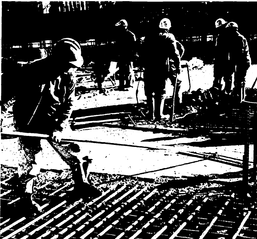
Cement masons must know their materials and be familiar with various chemical additives that speed or slow the setting time.
