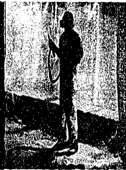
Ceiling asbestos wetted to decrease airborne fibers during removal process.
