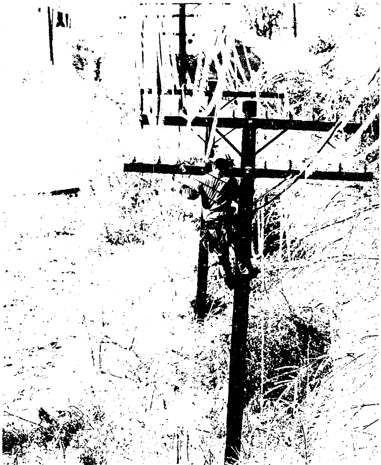
10E - A threat of severe winter storms causes millions of dollars damage each year to overhead transmission lines. Portland, Ore., December, 1977.
