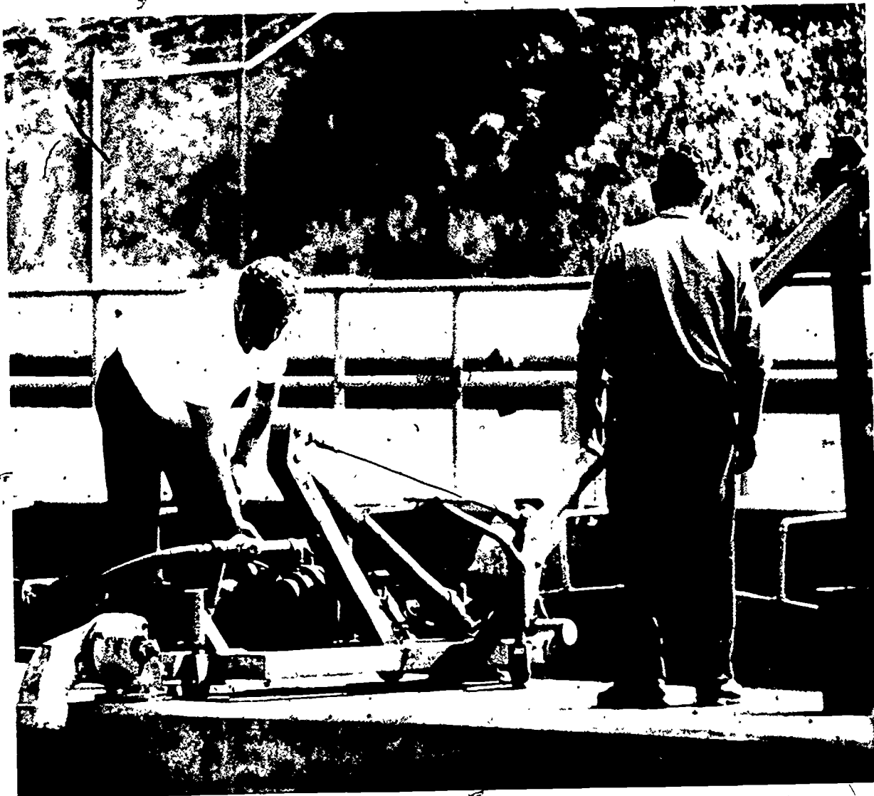
Plant maintenance must be performed on a routine, planned basis by qualified personnel.
