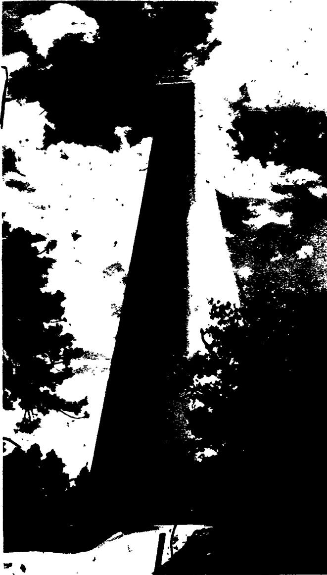
Solar physics. The 7-year-old Solar Vacuum Tower Telescope at Sacramento Peak Observatory in New Mexico provides critical data about solar flares, magnetic fields, and the velocities of matter in the solar atmosphere. Its 30-inch fused quartz entrance window is 136 feet above ground level, and the bottom of the evacuated optical system is 193 feet below ground.
