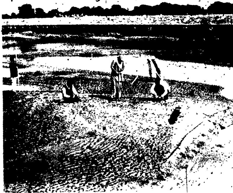
Water research. As part of a U.S.-Pakistan joint research project, scientists (left) meter the water surface level of a Link Canal and take a soil core (right) to determine particle size of bottom sediments. The Link Canals, built to redistribute scarce water among Pakistan's rivers, are part of one of the world's most ambitious water development projects. Their size and variety make them valuable for research on the design of modern irrigation channels. (Photos by Khalid Mahmood/George Washington University.)
