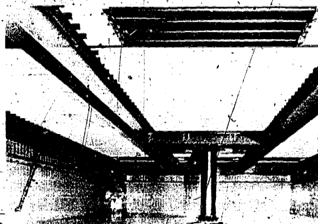
Swimming pools are constructed with two bottoms, one of which may be moved up and do - n to quickly change the depth of the water for different levels of swimming skills.
