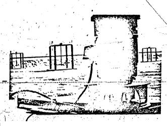
Twelve of these mechanical surface aerators will help to reduce the organic pollutants in the effluent.
