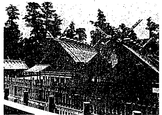
Side view of the Grand Shrine of Ise. The buildings are of Japanese cypress with occasional gold ornaments. This shrine has been rebuilt every twenty years or so for the past thirteen centuries.
