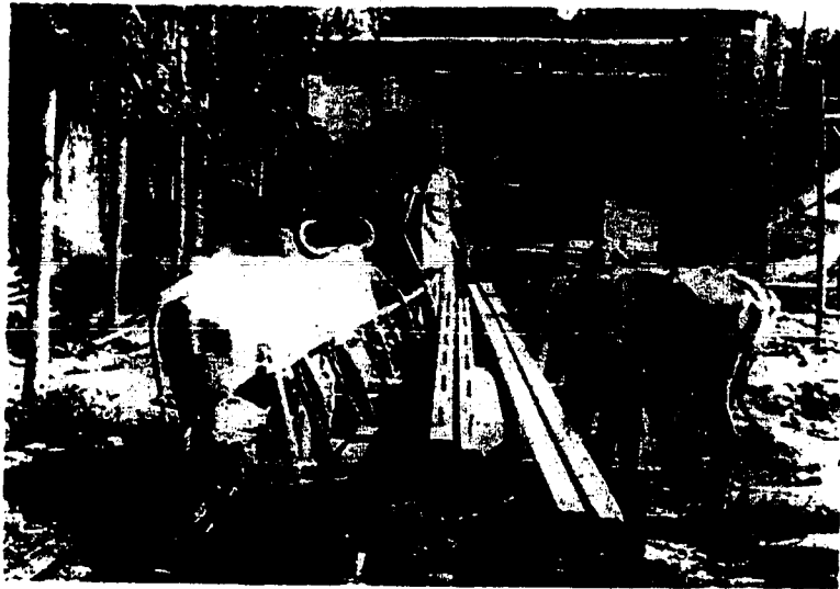
Plate 4. Building elements have to be designed for transport to the rural areas by whatever means is available - often, as in this case, by bullock cart.
