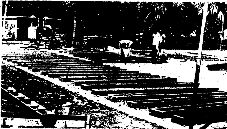
Plate 8. At the casting centres, only a concrete mixer and a vibrator are used to make the channels. All other work is manual, hence labour-intensive.
