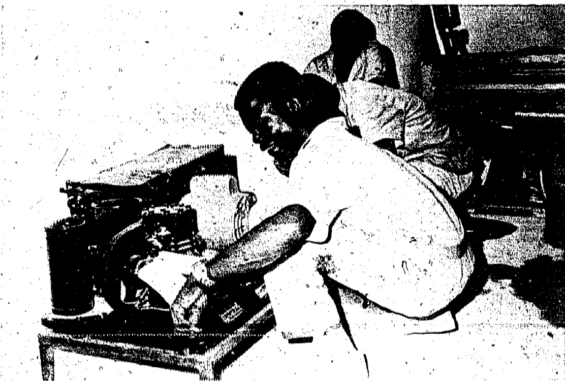
Compressor installation AID/ORT refrigeration and electromechanics training Center - Libreville
