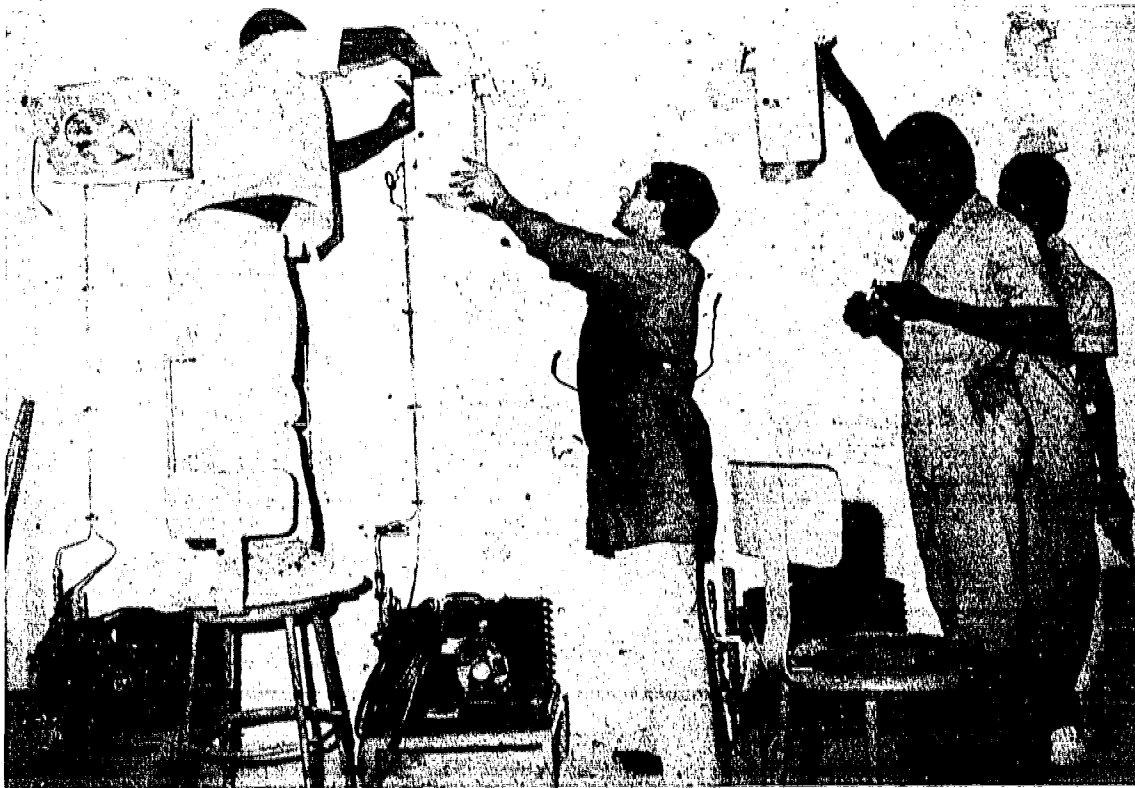
Compressor installation AID/ORT refrigeration and electromechanics training Center - Libreville
