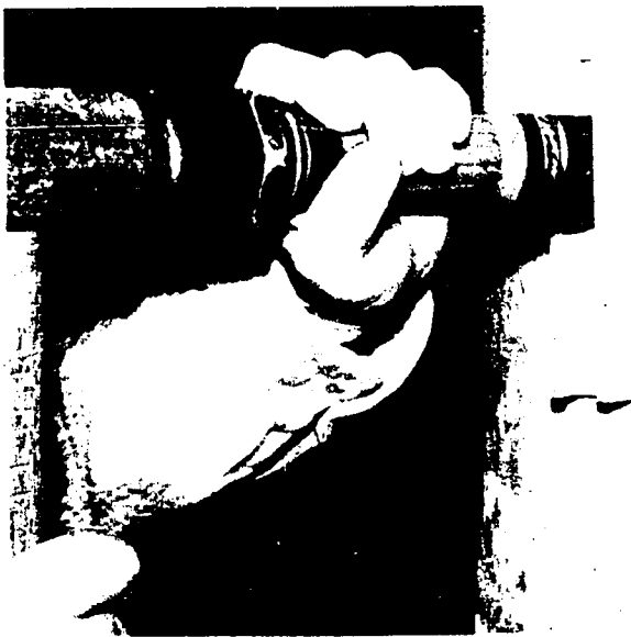
Figure 4-17.—Fastening channel to concrete.
