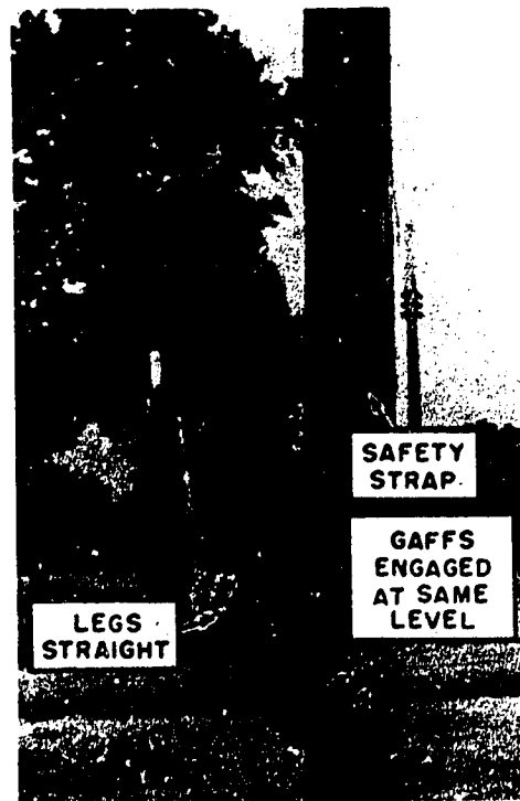
73.313 Figure 10-27.—Working position.
