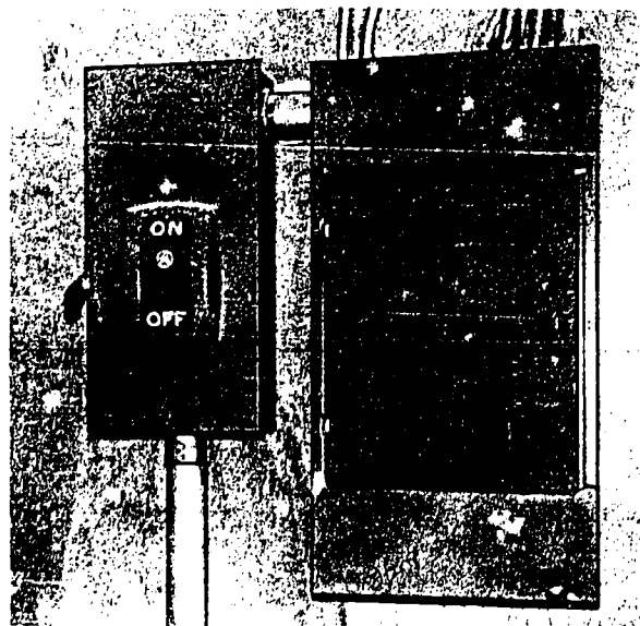
Figure 8-23.— Entrance switch marked to show open (OFF) and closed (ON) positions.
