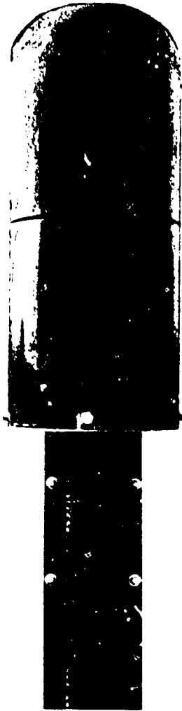
73.215 Figure 13-27.— Terminal housing with cover in place.
