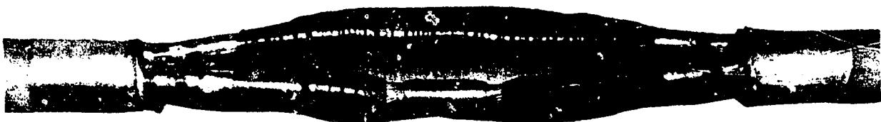
Figure 11-27. — Pouring compound.
