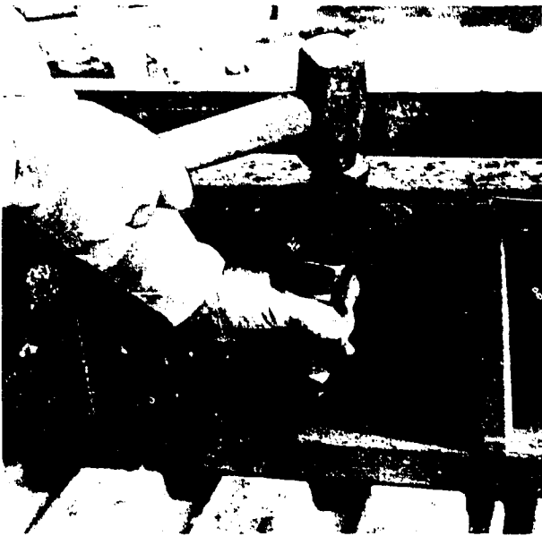
Figure 4-16.—Toenailing wood to hollow metal decking.
