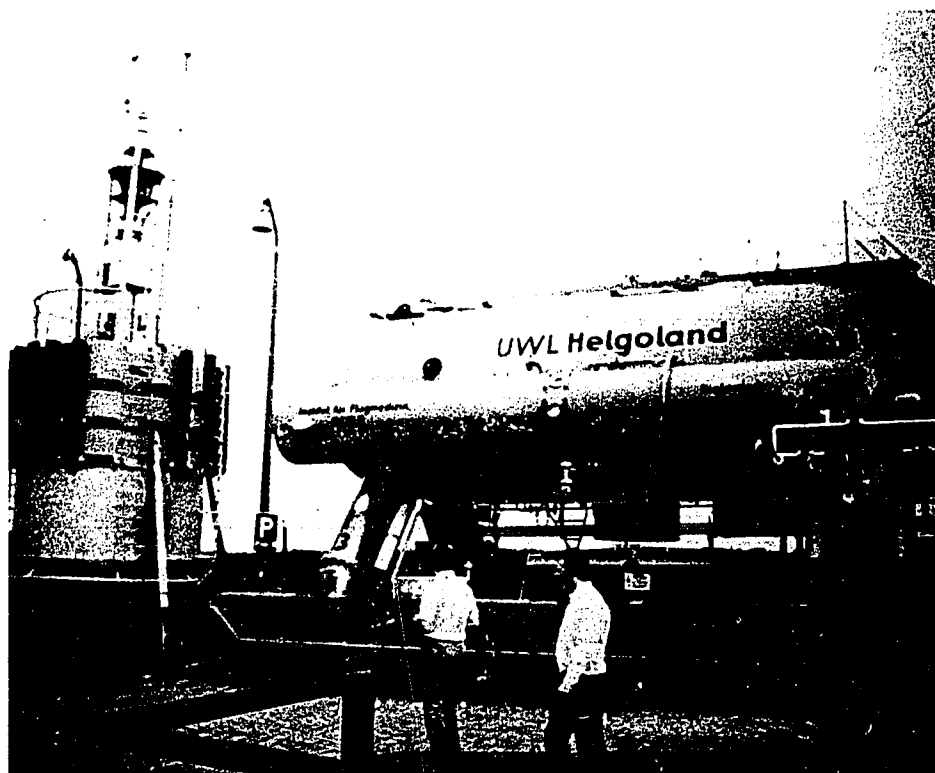
UWL HELGOLAND—Energy Buoy at Left. New Wet Room Attaches at Right
