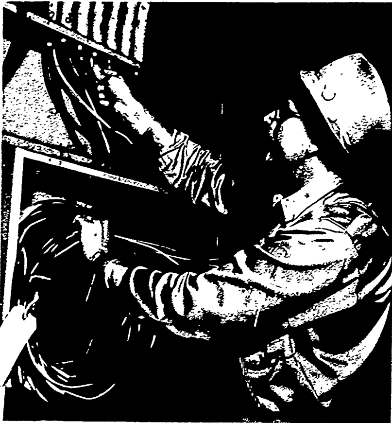
Electrician installs wiring.
