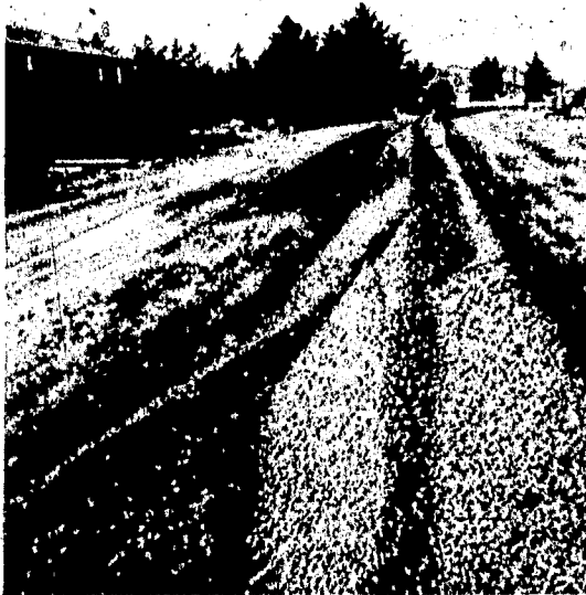
AGGREGATE AND ASPHALT WINDROWED IN THE MIDDLE OF THE STREET DURING THE MIXING PROCESS.
