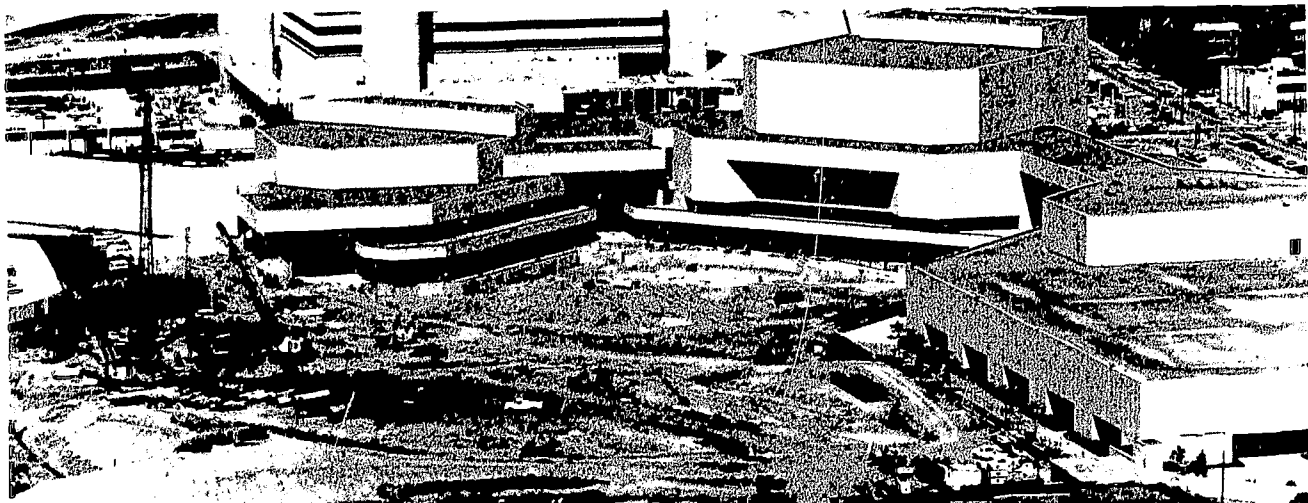
Site during construction
