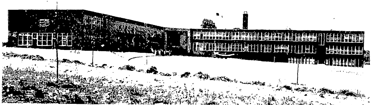
Exterior before rehabilitation
