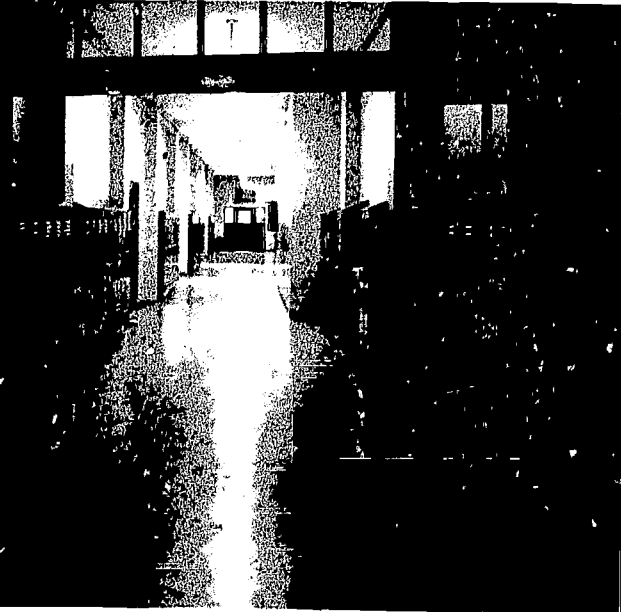
Corridor before rehabilitation
