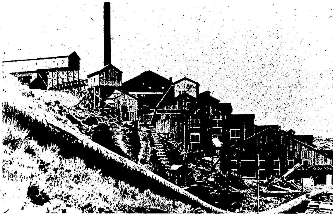
Fig.15. The Encampment Copper Smelter, 1907.
