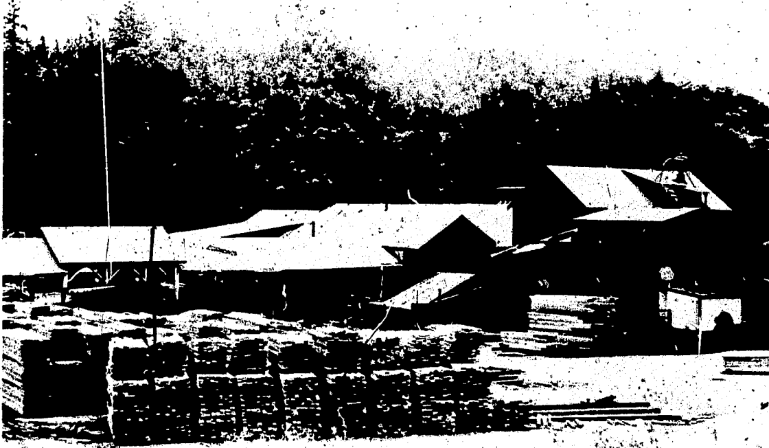
Fig.11, The Green Valley Lumber Co., Myrtle Creek, 1974. The only heavy industry in the South Umpqua School District.
