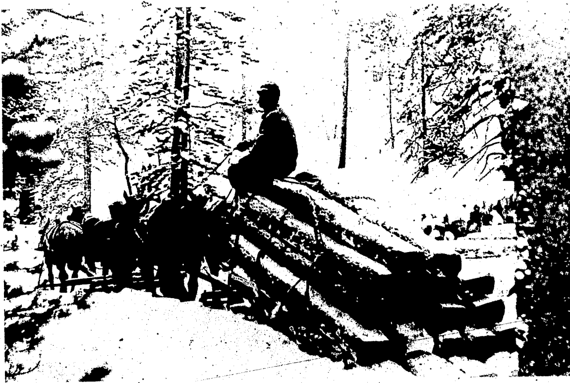
Fig. 8. Hauling fresh cut railroad ties on a "go-devil" near Encampment, Wyoming, c. 1908.
