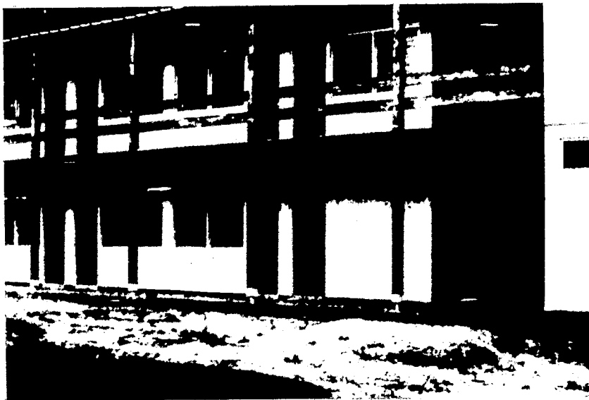
Fig. 2 A Modern Trend in Kenya Taita FIC with double storey dormitory block and built-in ablutions
