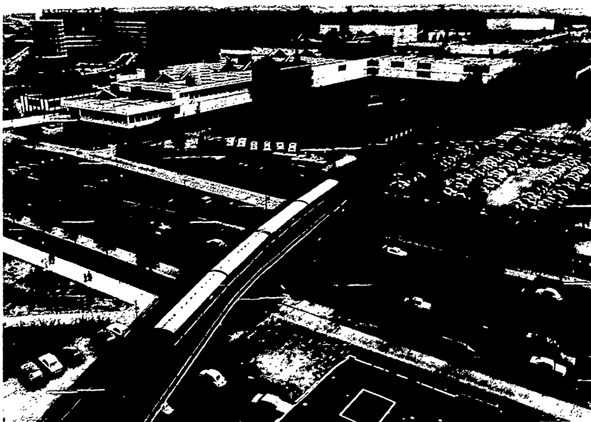
Photo IX - The Metro viaduct, Zuidplein, Rotterdam. The station on the right was originally the terminus of the 6 km long metro line which came into operation in 1968, linking the north of Rotterdam with the south. Zuidplein, with its metro and bus stations, car park, shopping centre and theatre, is Rotterdam's most important centre on the south side of the river. The new portion, all above ground level, takes the original line out to the satellite town of Hoogvliet, and was opened in 1974. The total length of the metro is now 17 km, 3 km being underground, under the city centre and the river.
