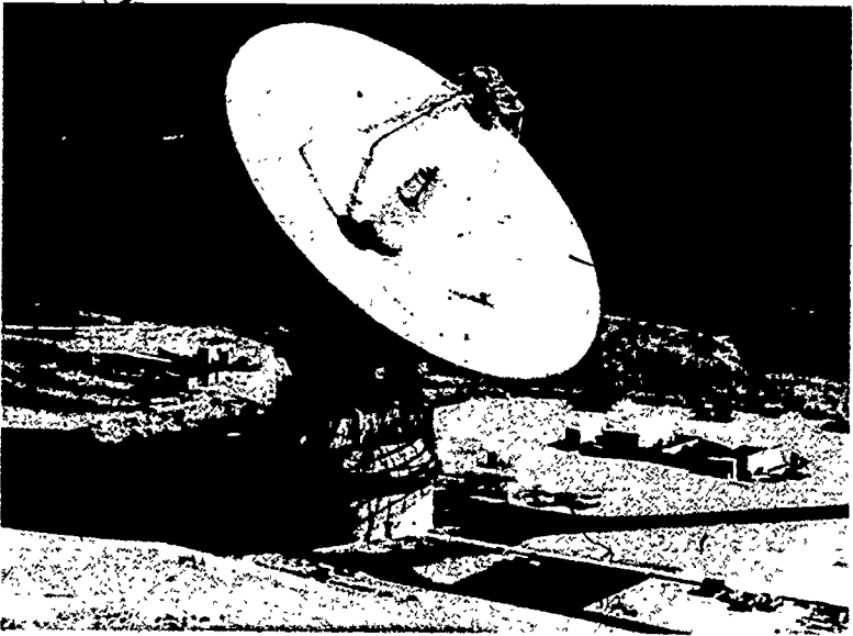
Figure 43. GIANT DISH ANTENNA. This is the 210-foot (in diameter) antenna at Goldstone, California. It is used for planetary probes and for communicating with the astronauts when they are on the moon or near it. Two similar giant antennas, one in Australia and the other in Spain, will be part of the NASA Deep Space Network.
