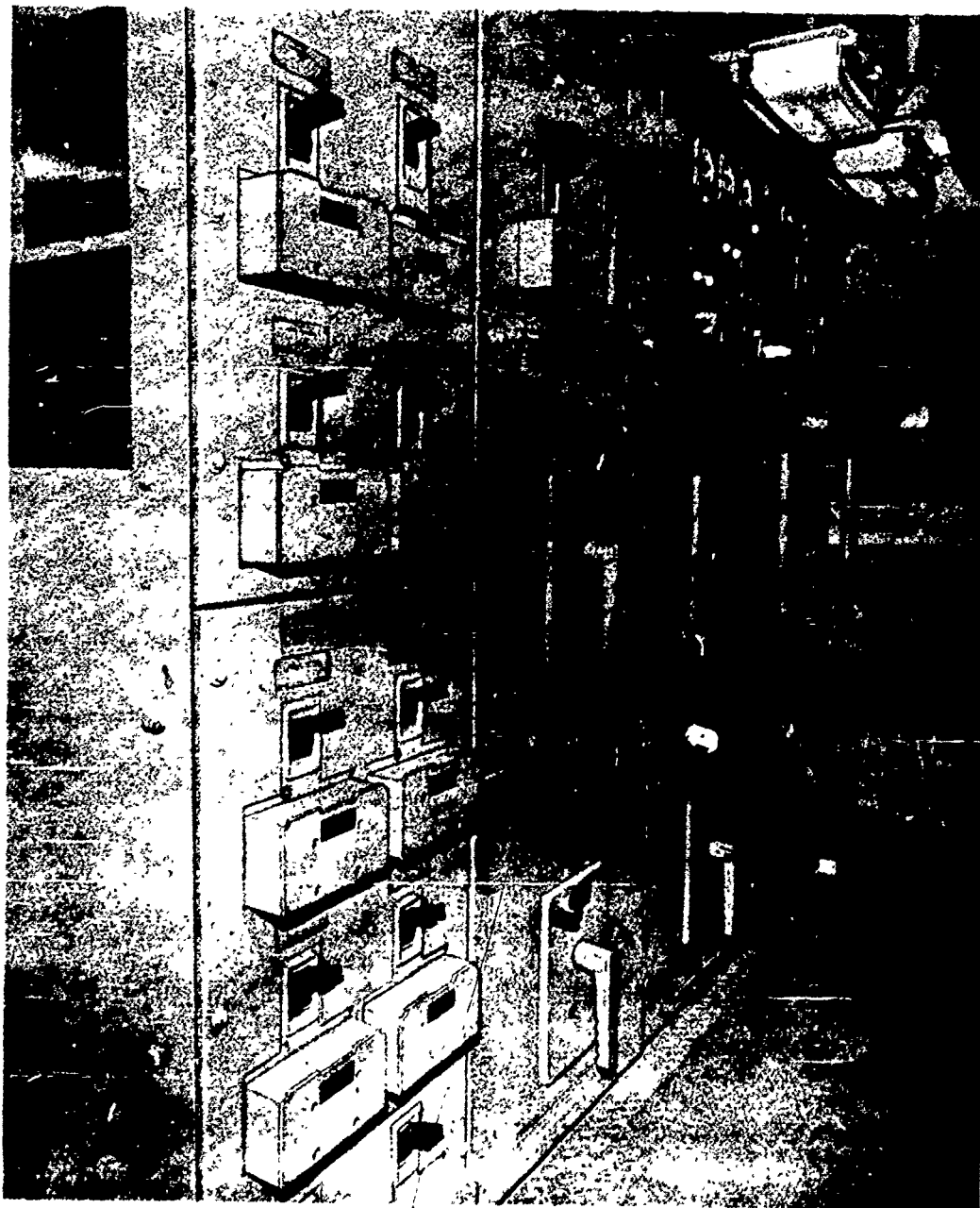
Figure 5-12.—Ship service switchgear No. 1S: section 1SA.
