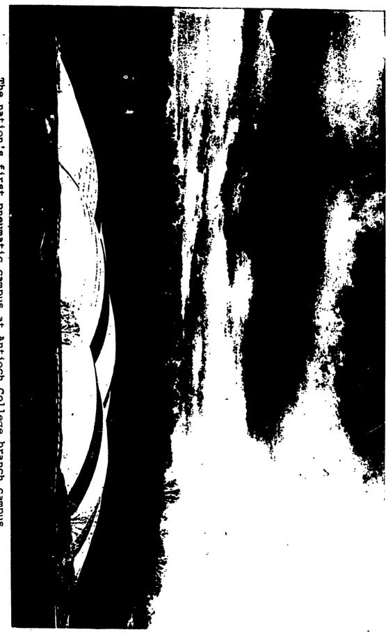
air pressure, covers an acre, enclosing portable classrooms, offices  $\widetilde{\phantom{a}}$ The nation's first pneumatic campus at Antioch College branch campus and studios. When the campus is no longer required the air will be in Columbia, Maryland. let out, the "building" rolled up, and the site returned to a meadow. The vinyl film structure, supported only by
