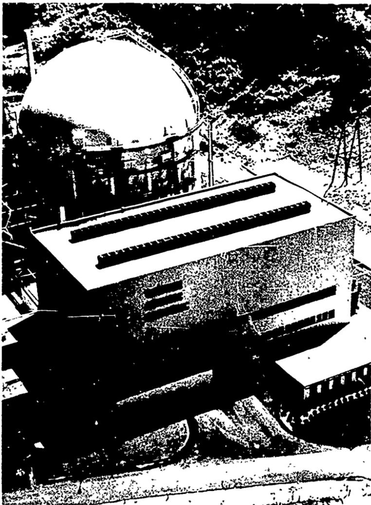
**Figure 19** *YANKEE Nuclear Power Station. Located at Rowe, Massachusetts, about 45 miles east of Albany, New York. Pressurized-water reactor, 175,000-net-electrical-kilowatt capacity, designed by Westinghouse Electric Corporation. Started commercial operation in 1961. Owned and operated by Yankee Atomic Electric Company. Yankee was the third large nuclear power plant to be built in the U. S.*
