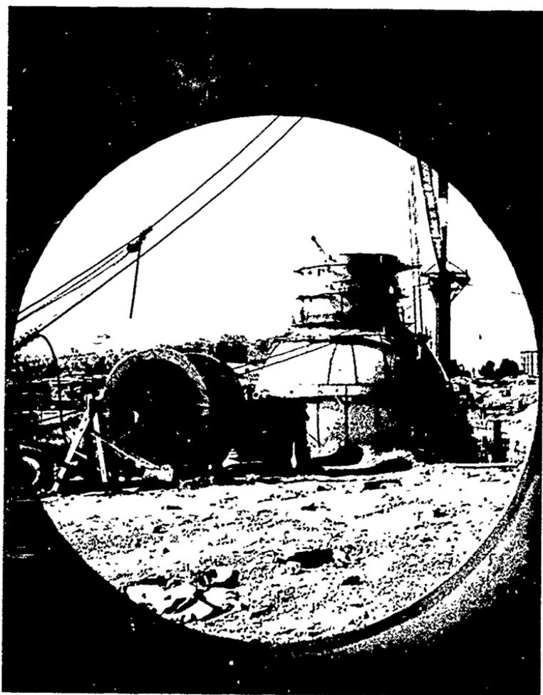
*Figure 31 NINE MILE POINT Nuclear Station, under construction. It takes several years time, a lot of material, and many hours of labor to erect a large power plant. In taking this picture, the photographer stood inside a large pipe that carries cooling water from Lake Ontario into the steam condenser. The huge, light-bulb-shaped steel shell in the foreground houses the reactor. A view of the finished plant is shown in Figure 32.*
