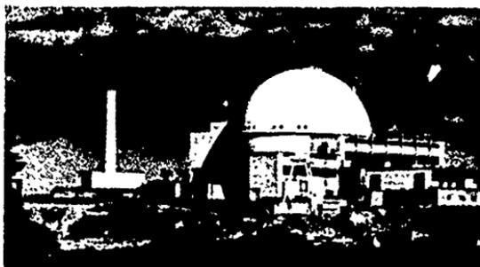
In addition to their work on gas-cooled reactors, the British are investigating other systems, including steam-generating heavy-water and liquid-metal-cooled breeder reactors. The Dounreay Fast Reactor, shown in Figure 36, is a 12,700-kilowatt experimental plant that has been in use since 1959. A new, 250,000-kilowatt prototype breeder reactor is located at the same site.
