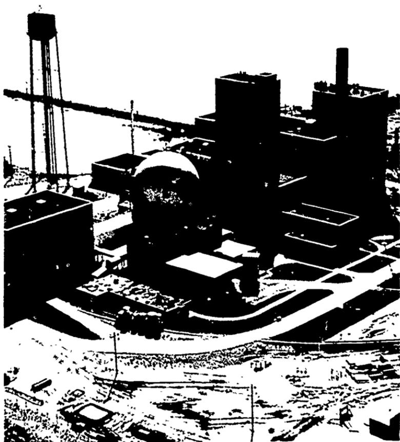
*Figure 21 ENRICO FERMI Atomic Power Plant. Located at Lagoona Beach on Lake Erie, near Monroe, Michigan, about 35 miles southwest of Detroit. Breeder reactor, cooled with liquid sodium, 60,900-net-electrical-kilowatt capacity, designed by Atomic Power Development Associates, Inc. Started power operation in 1963. Jointly owned and operated by Detroit Edison Company and Power Reactor Development Company. Enrico Fermi was the world's first large breeder nuclear power plant.*
