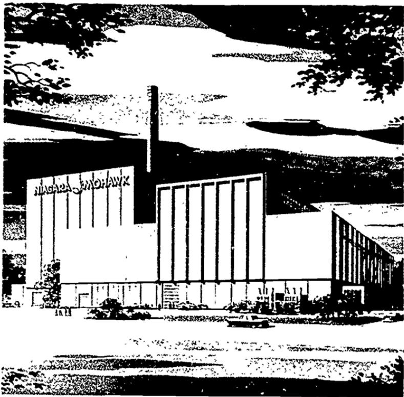
*Figure 32 NINE MILE POINT Nuclear Station. Located on Lake Ontario near Osuego, New York, about 35 miles north of Syracuse. Boiling-water reactor, 500,000-net-electrical-kilowatt capacity, designed by General Electric Company. Owned and operated by Niagara Mohawk Power Corporation.*
