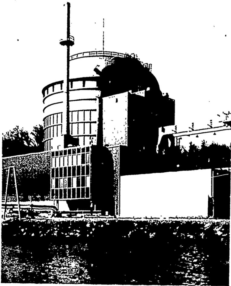
**Figure 23** PEACH BOTTOM Atomic Power Station Unit #1. Located on the Susquehanna River near Peach Bottom, Pennsylvania, about 65 miles southwest of Philadelphia. Helium-cooled reactor, 10,000-net-electrical-kilowatt capacity, designed by Gulf General Atomic. Started commercial operation in 1967. Operated by Philadelphia Electric Company, Peach Bottom is a demonstration reactor featuring high temperatures and a gaseous coolant. Units #2 and #3 are located at the same site.
