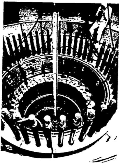
**Figure 41** The interior of the reactor vessel of the LINGEN Nuclear Power Station in West Germany. The inside diameter of the vessel is about 12 ft. This boiling-water reactor has been in operation since 1968.
