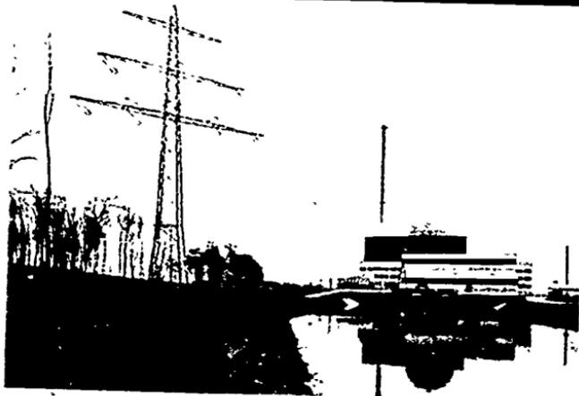
**Figure 40** West Germany's GÜNDREMMINGEN Nuclear Power Station. This 237,000-kilowatt plant was Germany's first large-scale nuclear power station. It uses a boiling-water reactor and has been in operation since 1966.
