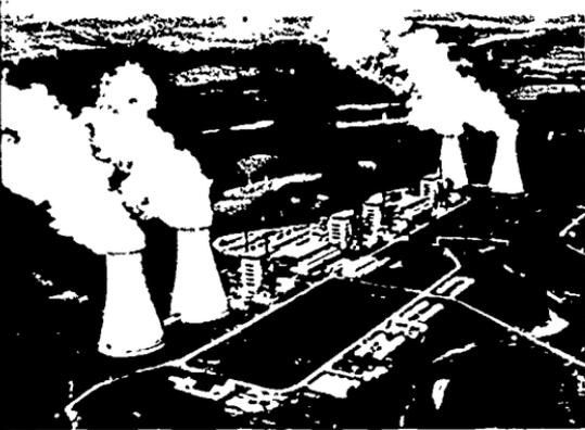
**Figure 34** England's CALDER HALL Nuclear Power Station. The tall structures are cooling towers, which are employed in locations where a large body of water is not accessible. These towers cool the condenser cooling water so that it can be used again, and they emit steam, not smoke. Four reactors supply steam to two turbines. Total capacity of the station is 198,000 electrical kilowatts.
