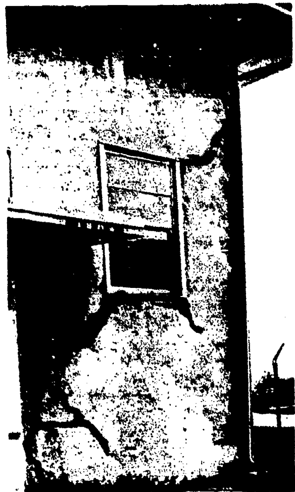
Figure 11-1. —Signs of foundation displacement.
