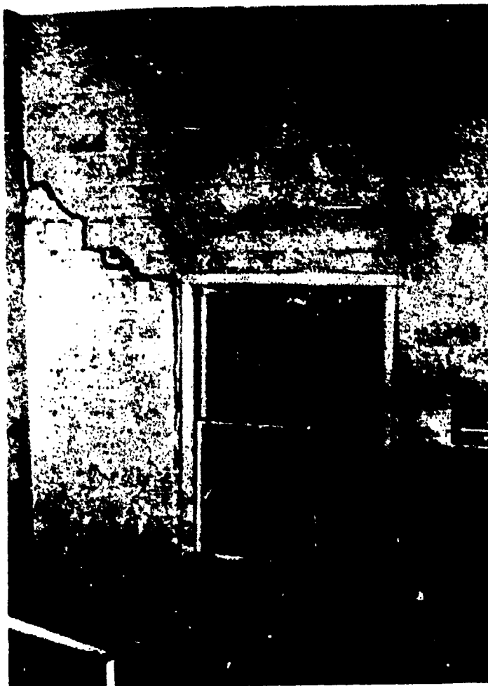
Figure 11-1. —Signs of foundation displacement.
