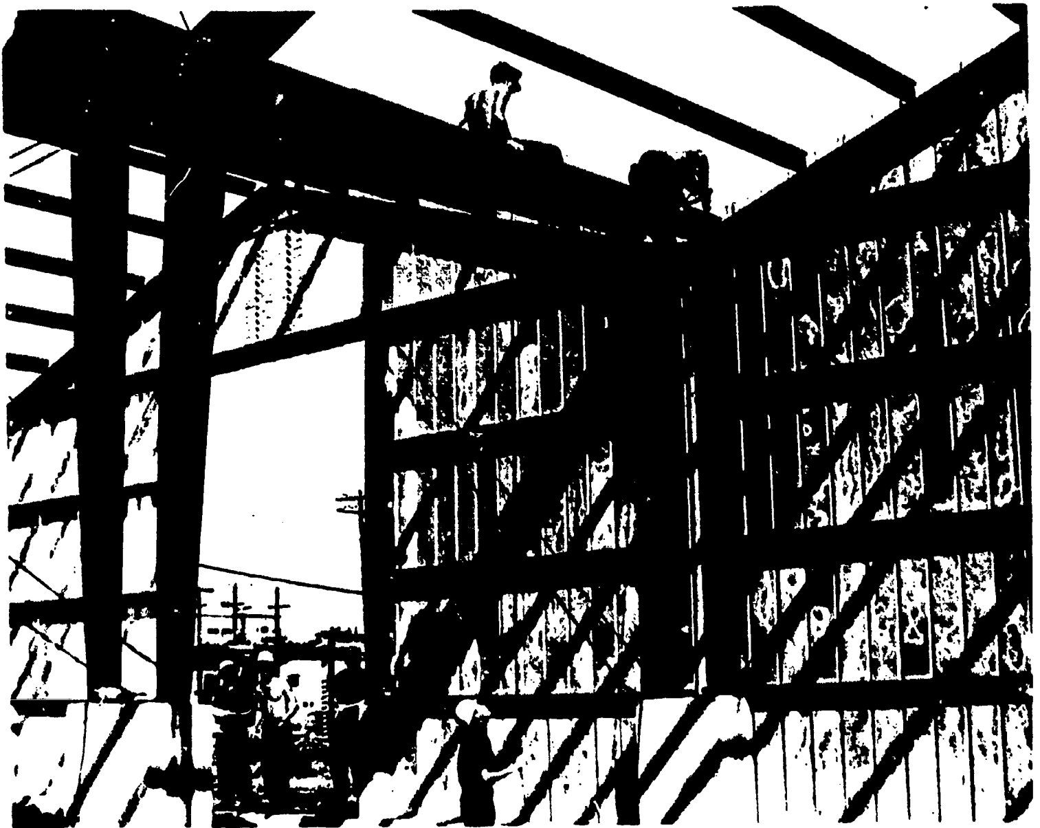
Figure 7-25. —Erecting Pascoe buildings side-by-side.
