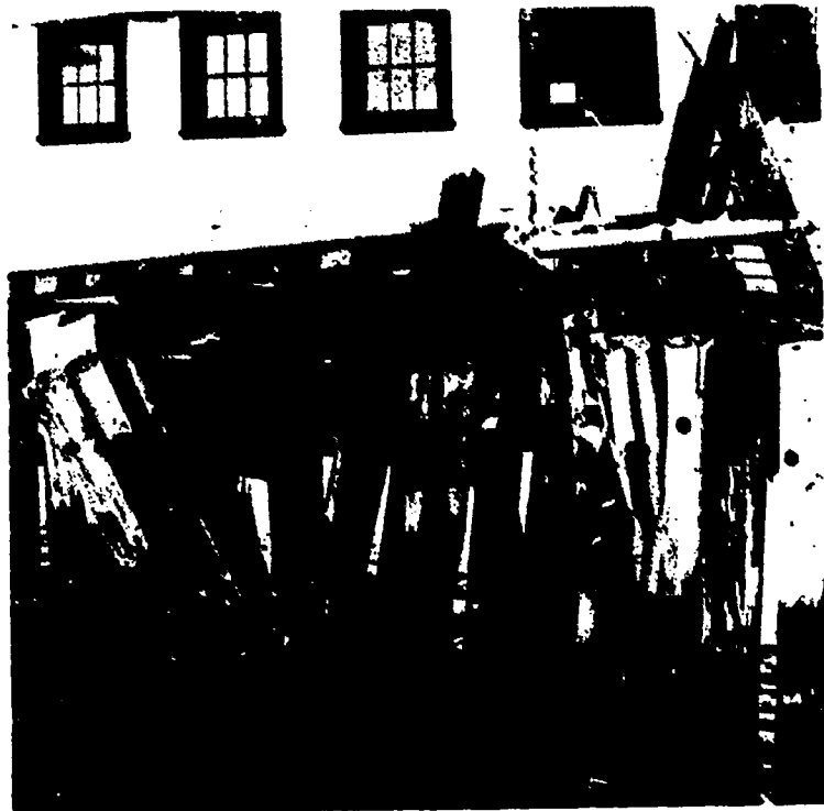
Figure 11-36. —Broken wooden piles.
