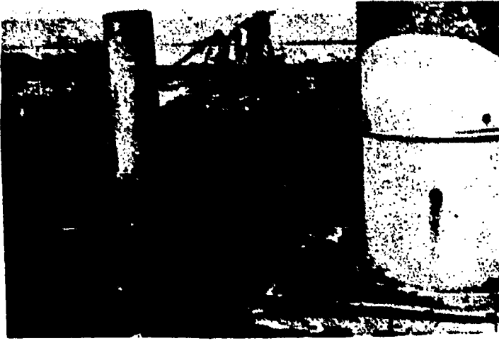
Figure 11-17. —Separation of metal flashing flange from roof—caused by exposed nails that have worked loose.
