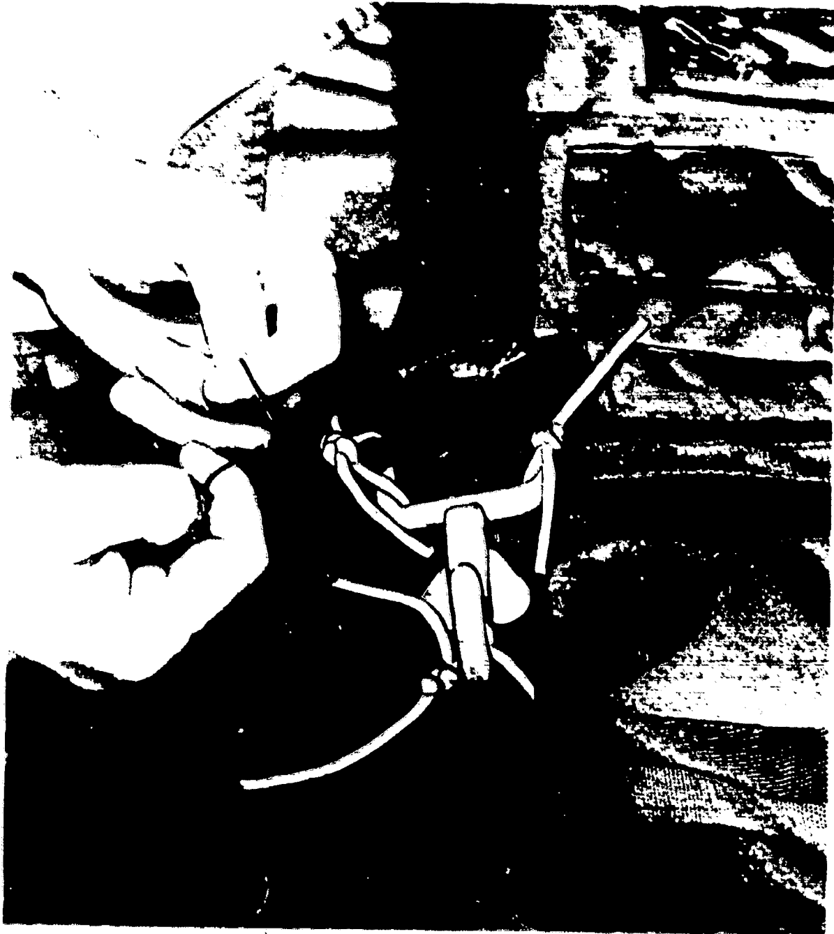
Figure 6-38.—Tying the riser assembly quick-disconnect snaps to the standard soft pack outer container.
