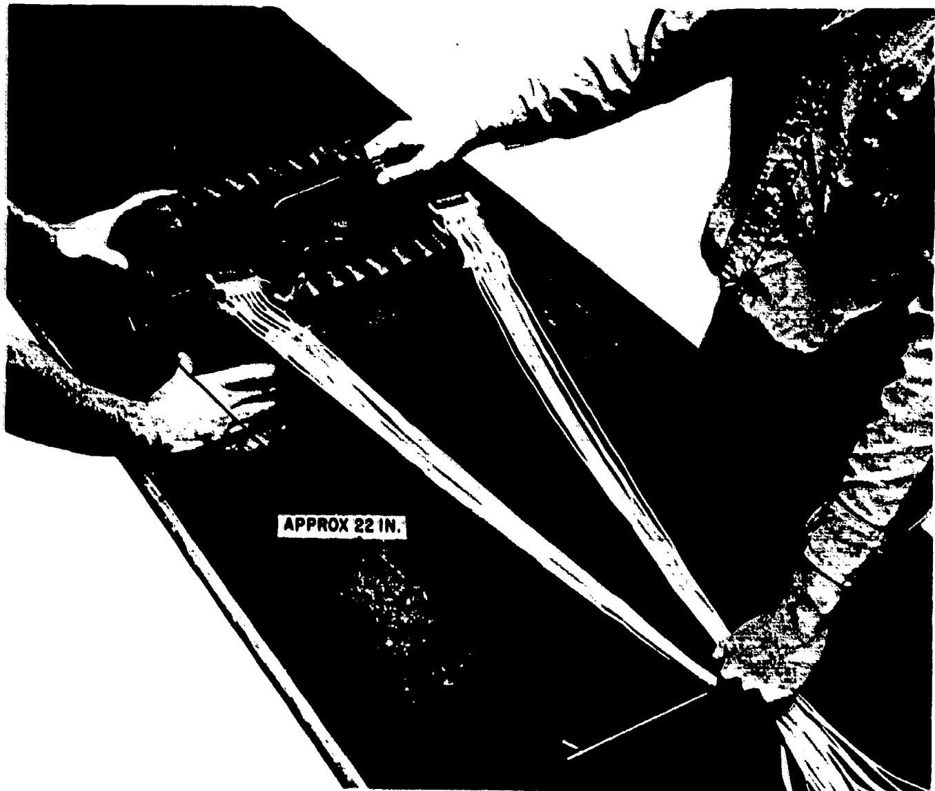
Figure 6-10.—Gaging length of suspension lines required for making first bight.
