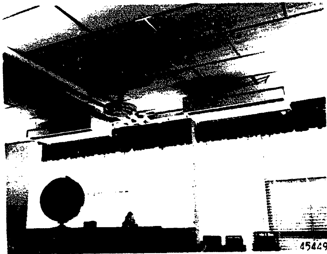
Ceiling Mounted Hot Water Convectors Added To Library to Provide Solar Heat
