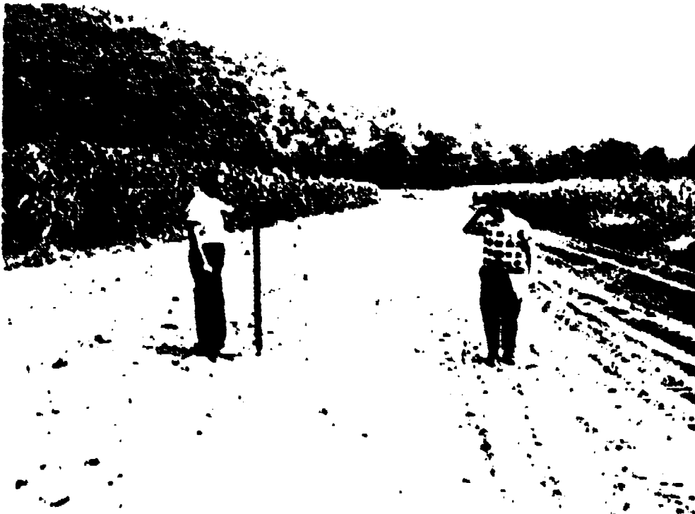
A Soil Conservation Aide assisting a Soil Conservation Technician determining the slope of a diversion ditch for water runoff control. Courtesy U.S.D.A. - Soil Conservation Service.
