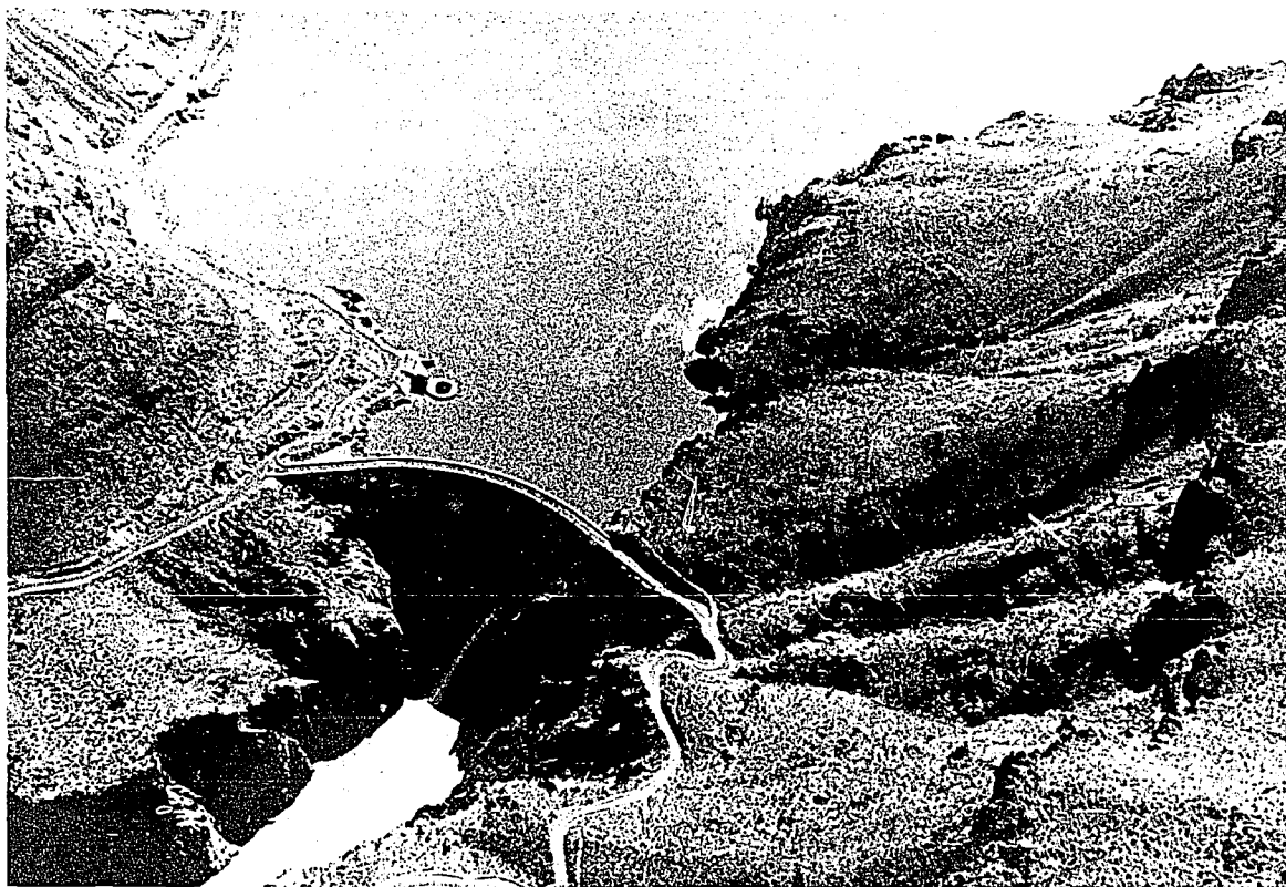
Figure 21. Owyhee Dam from the air. The abutments are against a body of rhyolite which has caused narrowing of the canyon here, creating an ideal place for a dam. The ring-like object is the gloryhole spillway.
