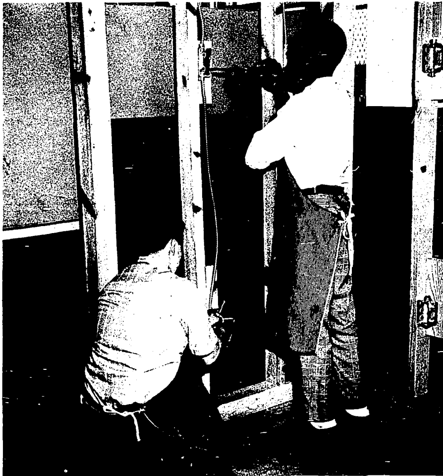
Students learn the fundamental skills of house wiring in a simulated frame structure.
