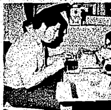
Operation of the tape-directed numerical control mill, which can be programmed to perform intricate jobs, is being learned by student in instructor Fred Gerinelli's class. The modern, $20,000 machine is found in many factories employing ROC graduates. Student (right), punches tape which programs drill.
