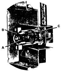
When not in use, this is the non-flowing condition of a gas outlet installed in hospital wall. Poppet "A" maintains gas seal, utilizing O-Ring "B". Valve body seal is maintained by O-Ring "C".
