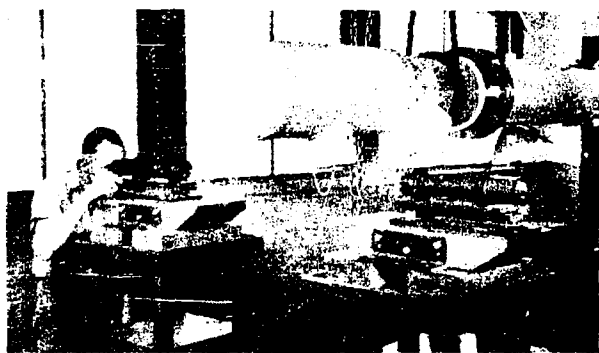
Figure 8-62.—Aligning the Mk 8 telescopes.
