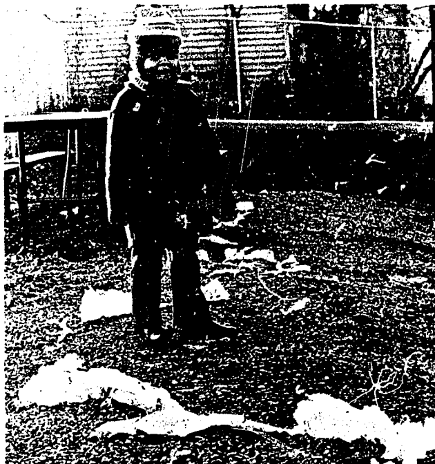
The edges of the polyethylene plastic work themselves up through the pea gravel.
