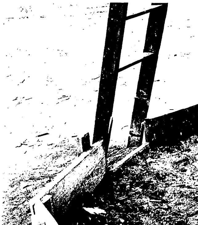
Splintered wood and a missing rung are dangers to an unsuspecting child.
