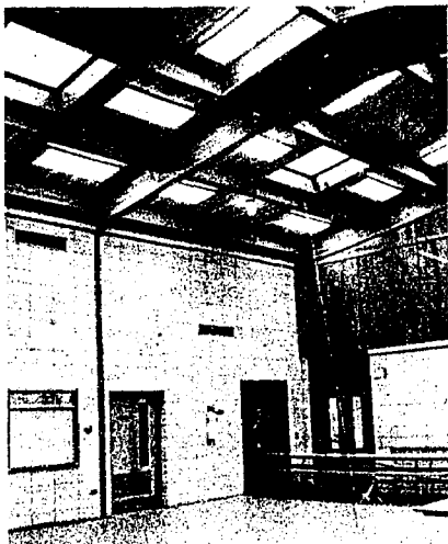
INAPPROPRIATE CEILING AND STRUCTURAL MATERIAL
