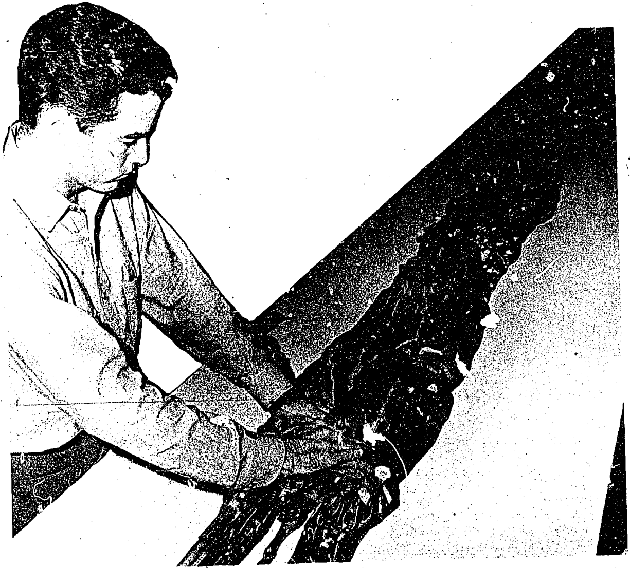
Figure 5-23.—Canopy folded to the width of the deployment bag.
