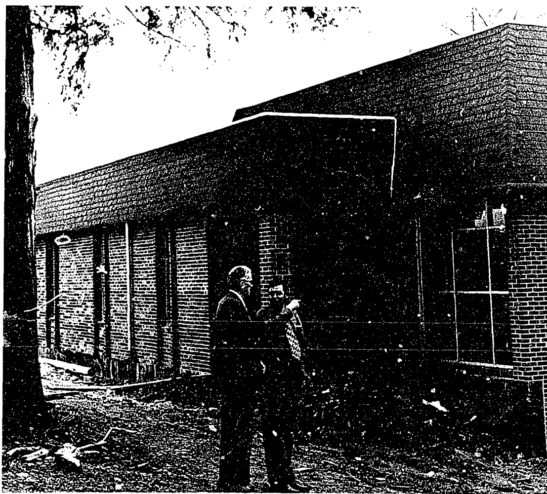
Lyle Donaldson, right, County Extension agent, shows L.J. Strickland, State Extension Community Development leader, the health clinic nearing completion in Pickett County, Tennessee. These two conducted a leadership training series which helped the community get started on self-improvement projects.
