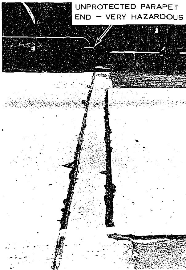
Figure 5-95. Sealed joints at bridge end between abutment backwall and adjacent deck and approach slab.
