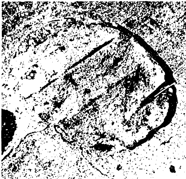
Figure 5-13. Large surface spall.
