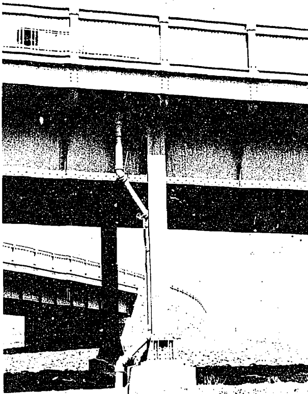
Figure 5-96. Deck drainage.
