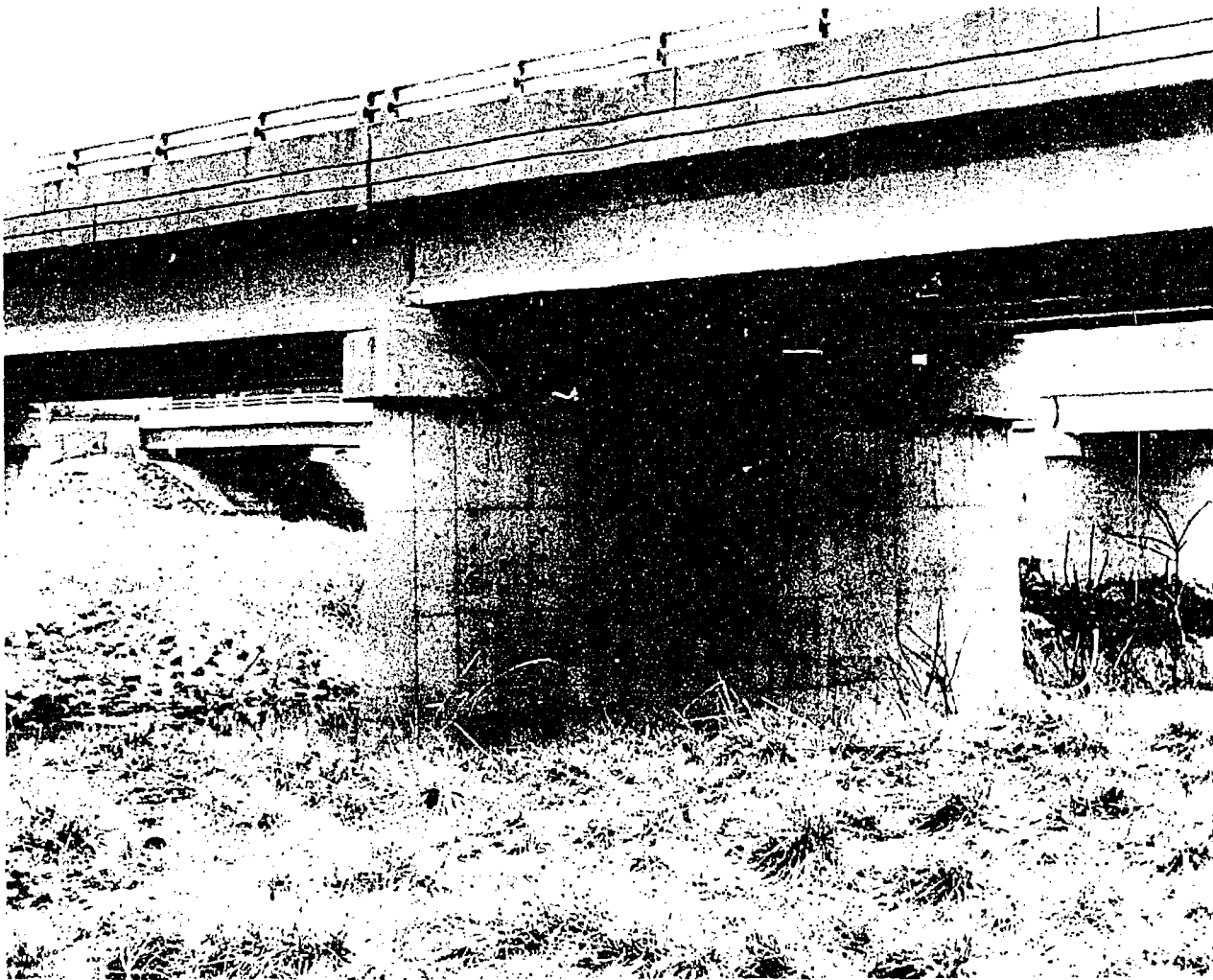
Figure 5-40. Solid concrete pier.
