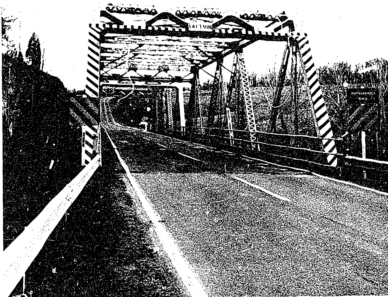
Figure 5-124. Approach to narrow bridge. Note paddle boards and striping of endposts and portal chord.
