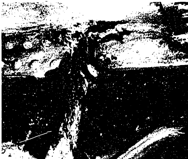
Figure 5-19. Rust on floor stringer. Note that web is completely rusted through.
