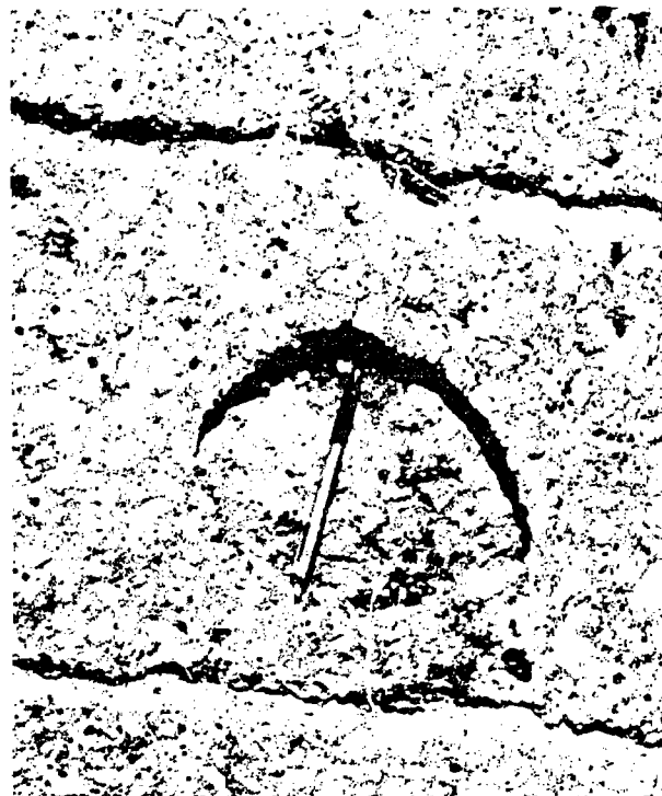
Figure 5-12. Small surface spall.
