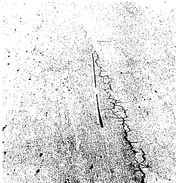
Figure 5-83. Longitudinal deck crack.
