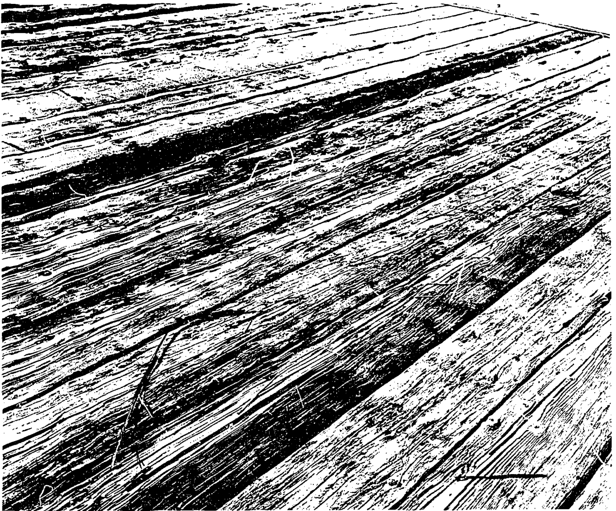
Figure 5-28. Weathering and wear of untreated timber deck.
