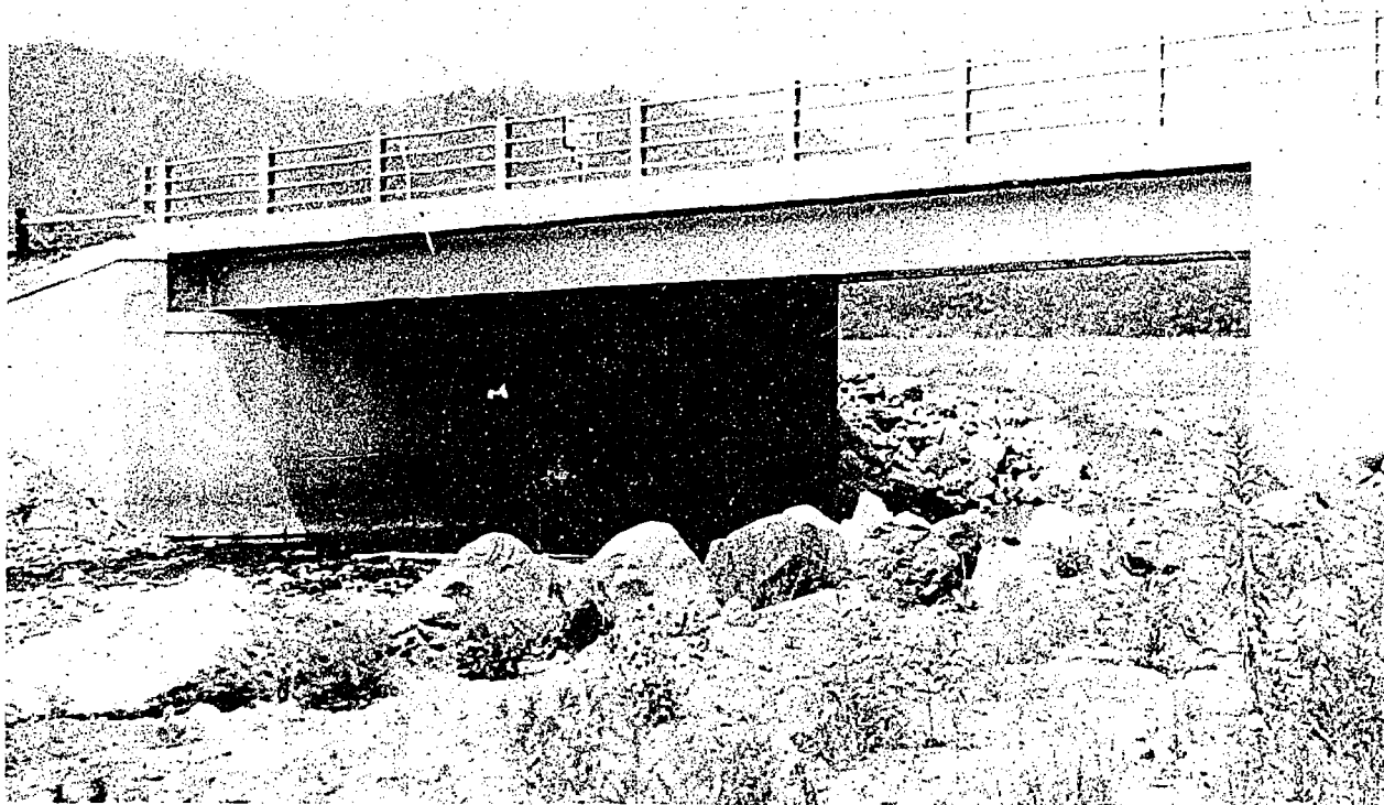
Figure 5-37. Full-height concrete abutment.
