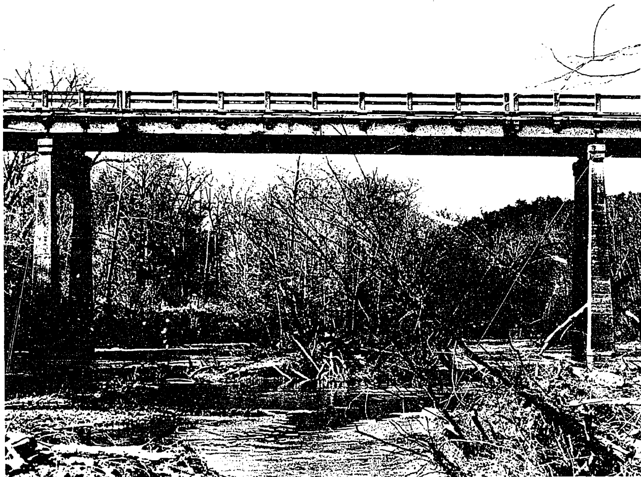
Figure 5-105. Drift and debris deposited in channel following flood.
