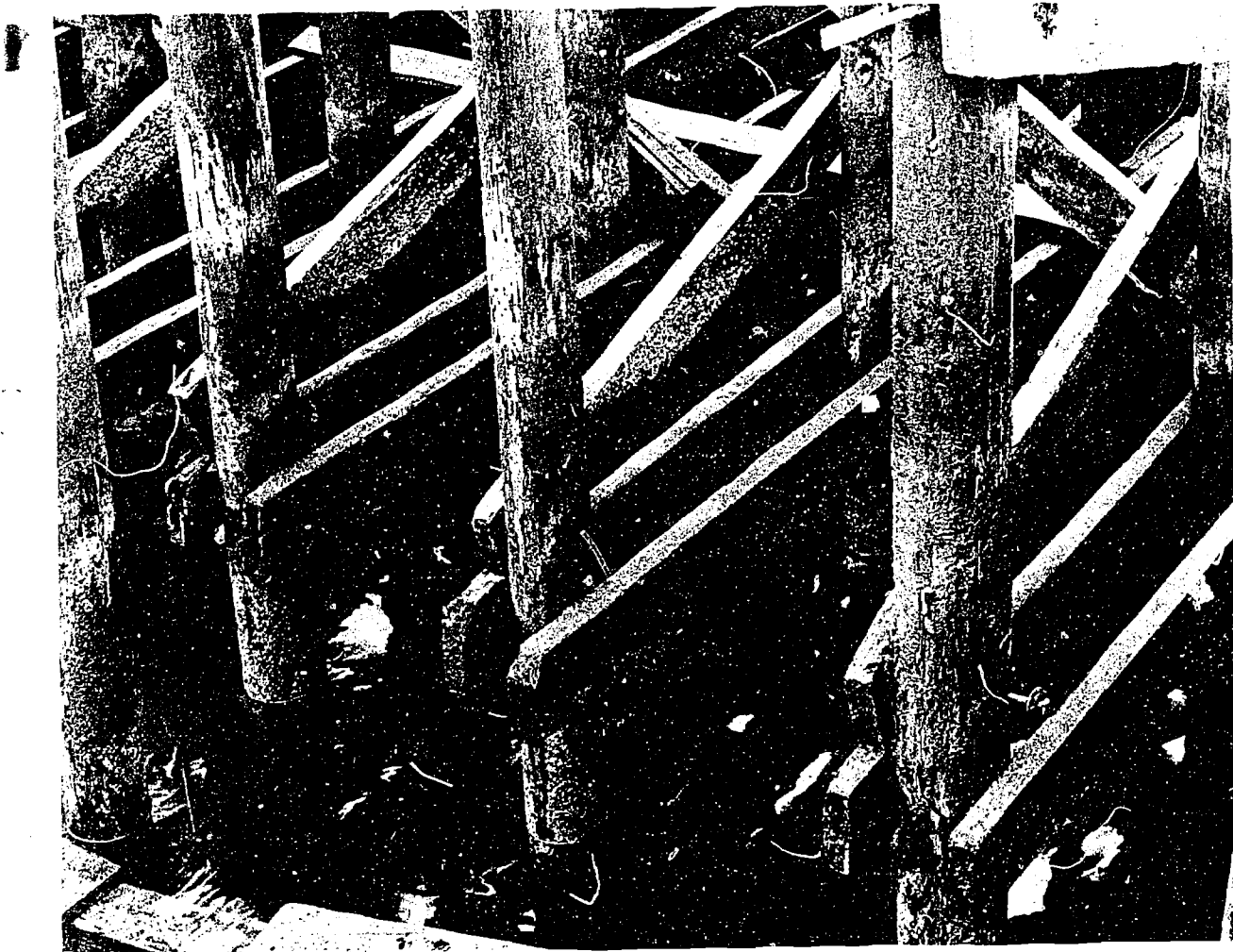
Figure 5-27. Limnoria attack in tidal zone. Attack began at cut off ends of bracing and progressed through bolt holes into piling.
