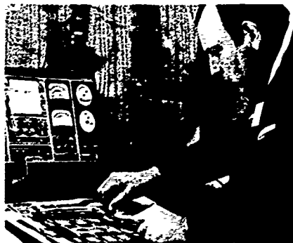
Vernon Williams checks an ignition wiring board in the mobile unit.
