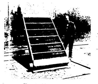
Figure 9. Solar air heater.
