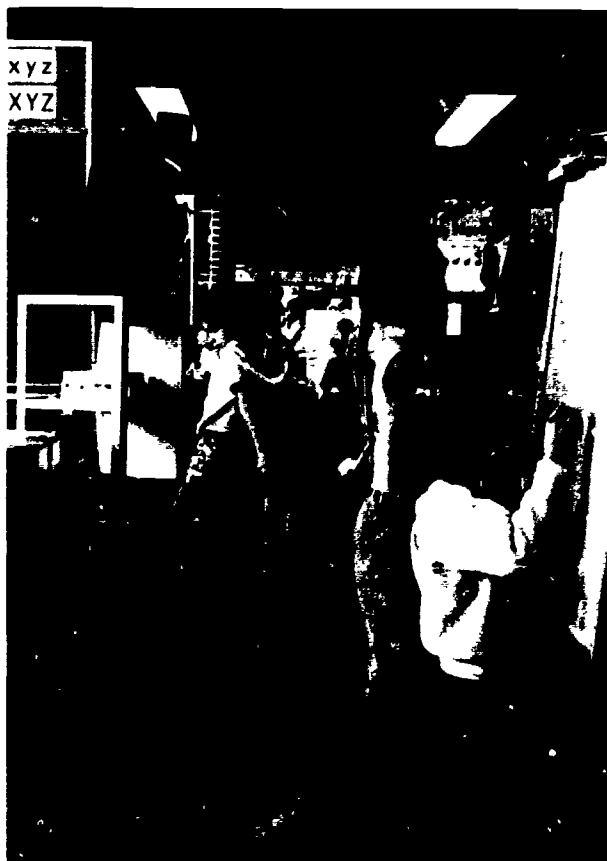
Walls were torn down in an old school building to create an open classroom.
