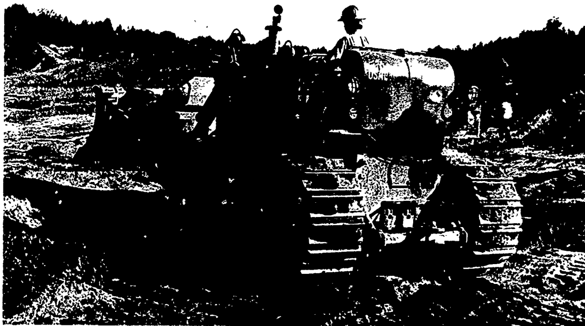
An MDTA trainee moves bulldozer into correct position. Note use of Federal excess property for the project.
