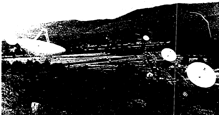
The three major telescope systems at the Greenbank, W.Va., site of the National Radio Astronomy Observatory are an interferometer array of three 85-foot-diameter telescopes, a newly surfaced 300-foot telescope that moves in a meridian plane (left, front), and a fully steerable 140-foot telescope (rear). (Photo by NRAO)
