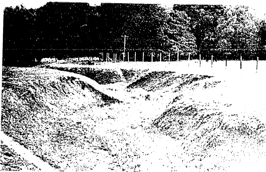
"Typical views of the drainage ditch ..."
