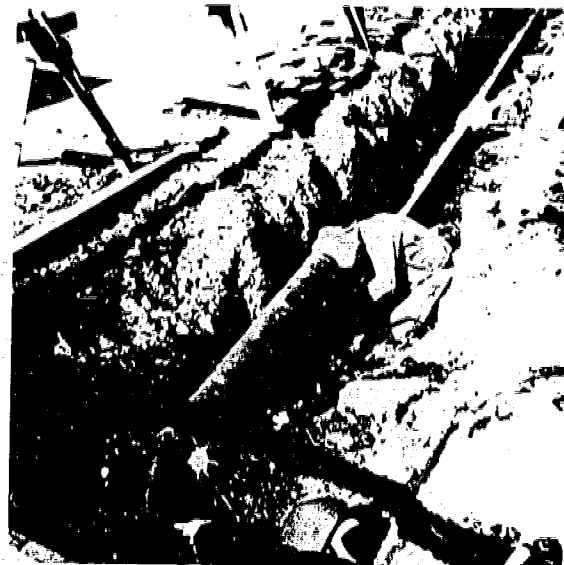
FIGURE 4: Repairing Buried Condensate Lines.
