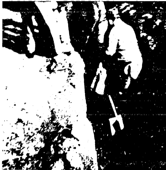
FIGURE 6: Insulating Backfill Type Coating Being Applied to Heating Piping. Coatings, alone, should not be relied upon to control corrosion.
