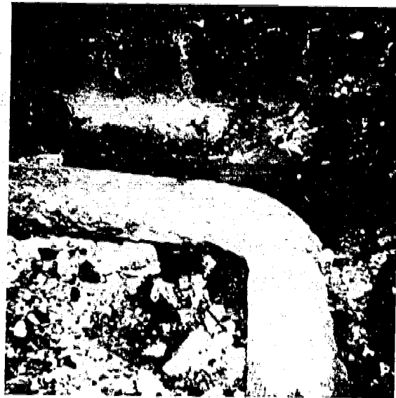
FIGURE 2: Corroded Steam and Condensate Piping.
