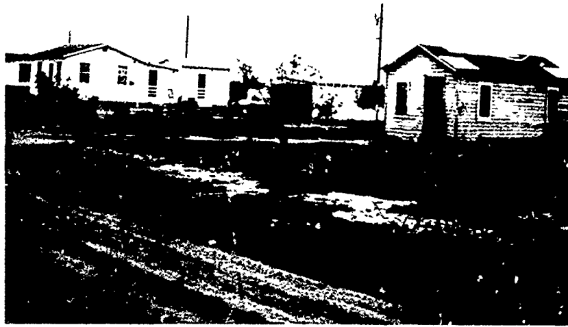
Migrant houses near Weslaco labor camp. One of the better houses is at the left.
