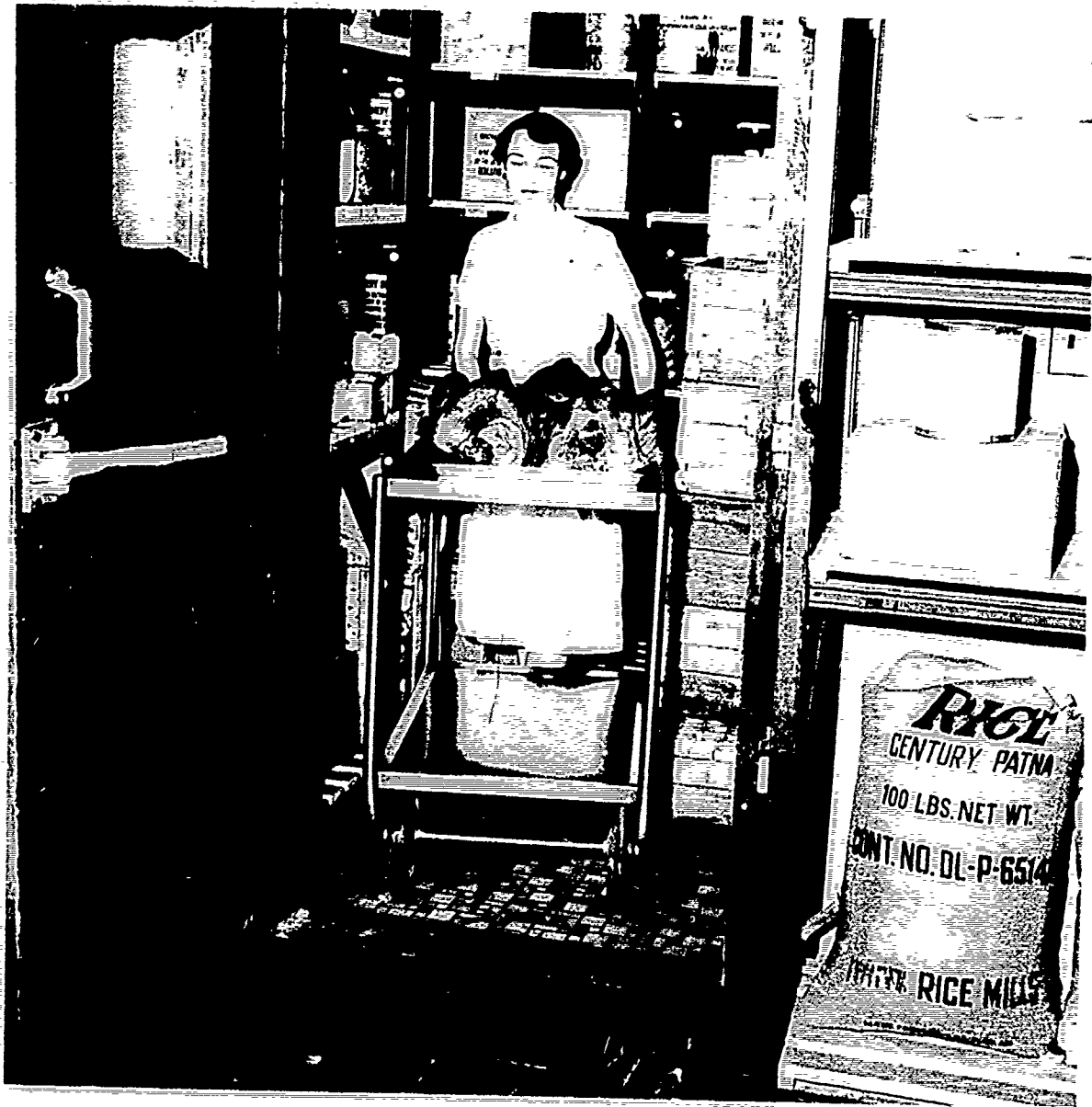
FIGURE 18.—Built-in walk-in refrigerator showing flush floor entrance.
