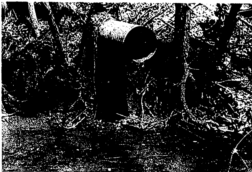
Sewage overflow outlet. Spring Creek on the grounds of the OEEC.
