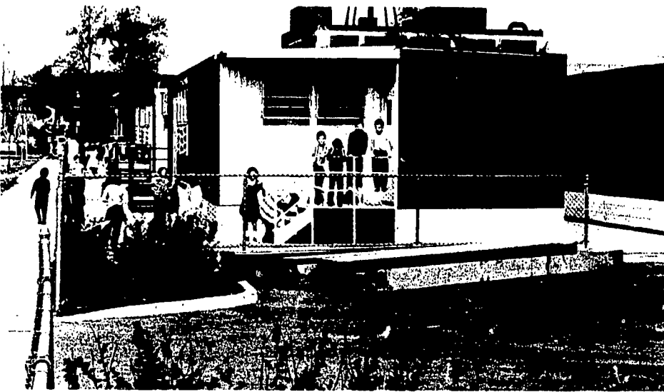
6 Staggered alignment of building sections allows for recessed steps and covered entry.
