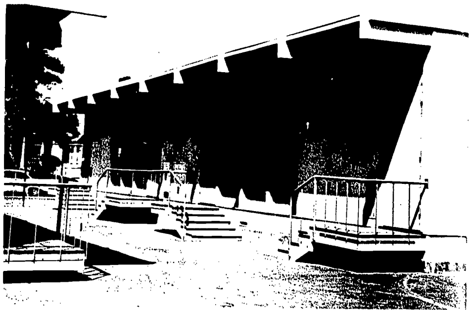
Basic Los Angeles portable classrooms (doubles) are stud frame with plaster stucco on wire mesh (no sidewall insulation) and plywood interior, 869ft 2 per classroom. Insulation is in roof structure. Portable toilet buildings (right) may include storage and janitorial space.
