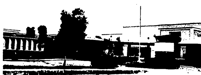
To relieve overcrowding of the main building . . .
