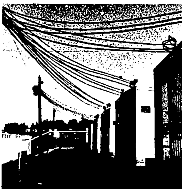
Codes allow overhead power lines—less expensive than trenched leads.
