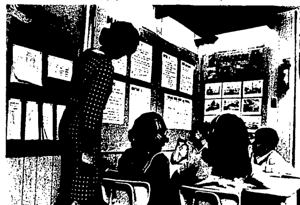
9-10 Lighted tackboard-display walls are overlaid on doors to supply closets and furnace space.
